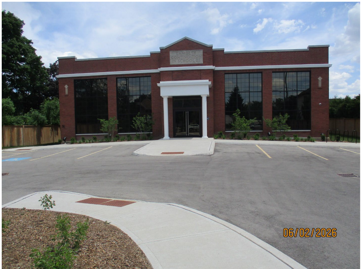
Image 1: Showing the completed rehabilitation of the former Lambeth Continuation School/M.B. McEachren School on the property at 4402 Colonel Talbot Road.
