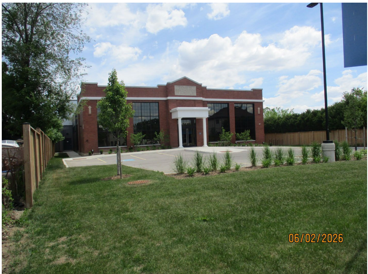
Image 2: Showing the completed rehabilitation of the former Lambeth Continuation School/M.B. McEachren School on the property at 4402 Colonel Talbot Road. Note, the medical and wellness centre addition is located at the rear of the building.
